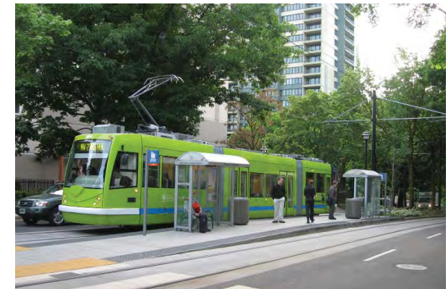
Median boarding provides for greater flexibility for curb lanes, which could be used for bike lanes, parking, additional landscaping, or for flex space activities such as outdoor dining.
