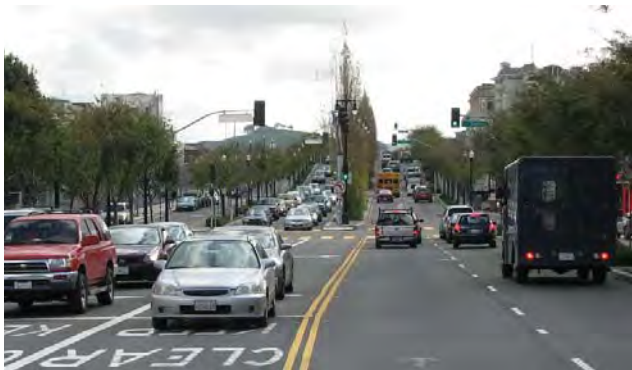
Narrow travel lanes on larger boulevards can still accommodate high traffic volumes at reasonable speeds suitable to an urban environment.
