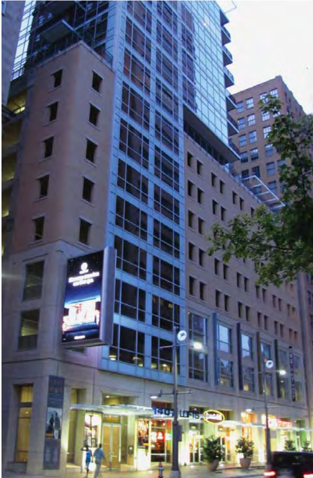
Much of the recent residential development in the CBD and surrounding districts has been focused on high-rise rental units, which have added thousands of residents to the Downtown area.
