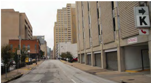
The parking experience for many is often unwelcoming, outdated and desolate, fueling perceptions about the desirability and safety of parking in Downtown.
